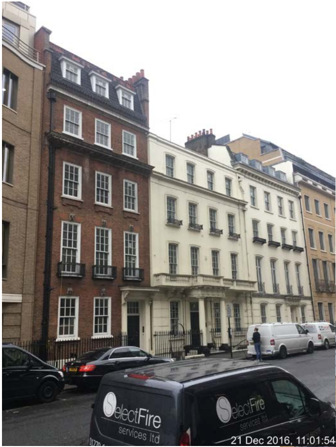
View of Grosvenor Street frontages (Top). View of Grosvenor Hill frontage (Bottom)
